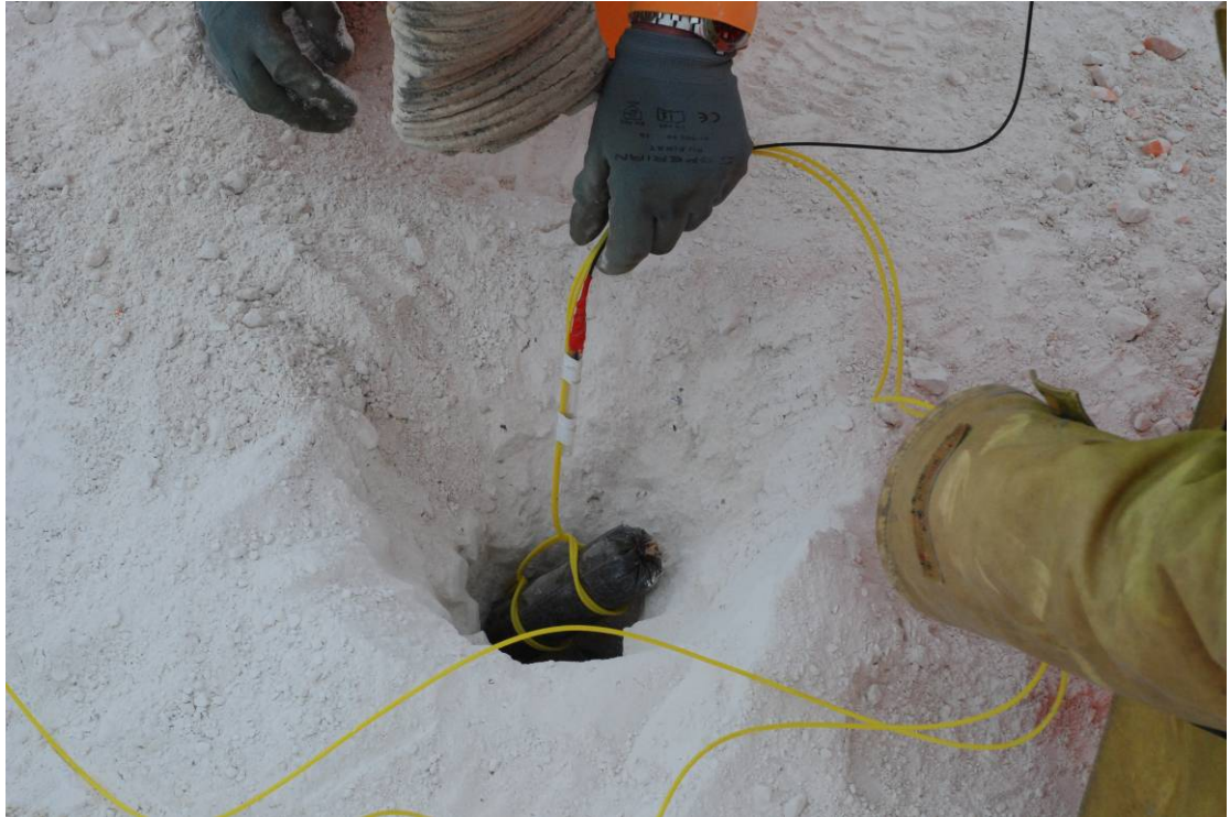
Plate 5.5. Lowering primer cartridge with Shock tube detonators and Optic fibre cable down the blast hole
